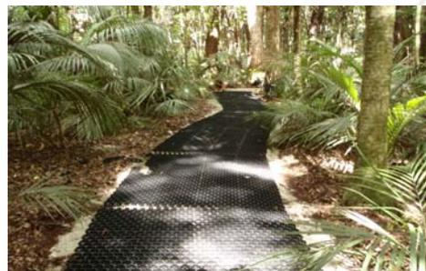
5. The mats were filled and compacted, using a local aggregate (Matakoitoki Red Rock)
