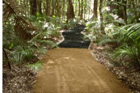
6. A cap layer was then applied of GAP20 with a small amount of cement added to aid compaction and surface strength.
